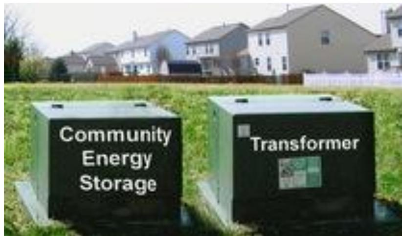
**Figure 7 : CES device next to a standard pad top transformer [53].**
